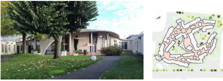
Figure 1: Photo of the Orb Pavilion, showing the garden view toward the refectory from the entrance. The single-story building envelops the garden. Noteworthy features include the concrete veil overhanging from the roof to the terrace. The facades feature numerous windows, from seat height in the bedrooms to full height in the refectory. Source: (Marie Tesson 2022). Figure 2: The Orb Pavilion floor plan shows an H-shaped building where every area connects to the garden or a terrace. Instead of corridors, it has a continuous agora that expands and contracts, punctuated by technical boxes. Source: (Marie Tesson 2024)
